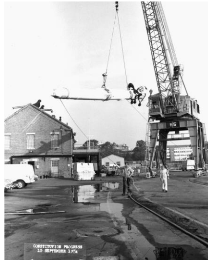
Constitution bowsprit with Portal Crane 65, September, 1974
