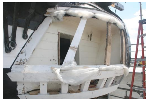
New framing for port quarter gallery, June 2016 13
