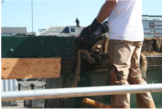
Removal of upper bulwarks at spar deck cap rail
