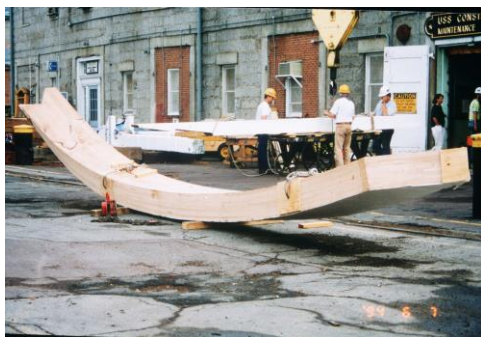
1992 restoration diagonal rider made from laminated white oak, before installation, 1994
