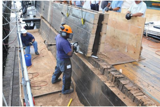
Antwine Burdett removes portion of starboard solid waist bulwarks; Eric Boyer looks on (left)
