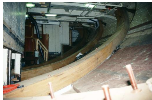
1992 restoration laminated diagonal riders installed in Constitution ’s hold, 1994
